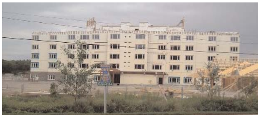
VBUCK®, Formtech and Hardi Wall installation in Ontario, Canada.
