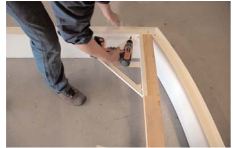
Brace using spreader and VBRACE™.
