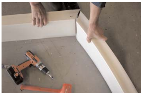
Fasten variable corners and join arch and strut pieces.
