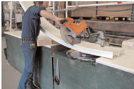
Cut angles with sliding miter saw.
