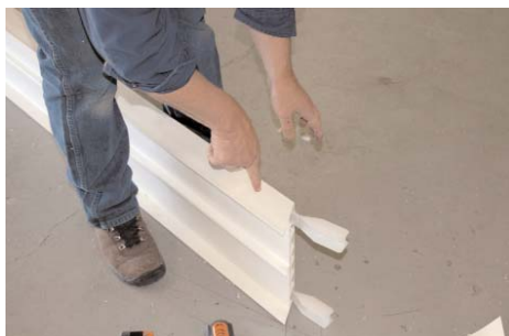
Plane and insert variable corners.
