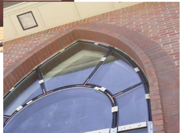
Each section of the curtain wall is attached to clips which are fastened through the VBUCK®, cellular PVC then into the concrete.
